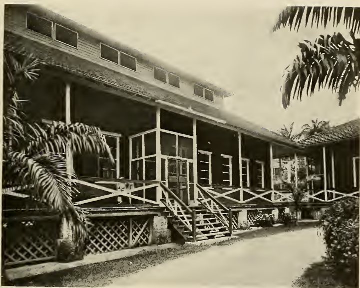
Old yellow fever ward at Ancon Hospital.
